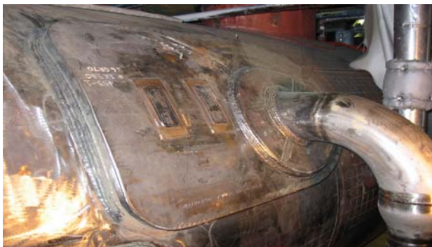
Installed Split PMCap
